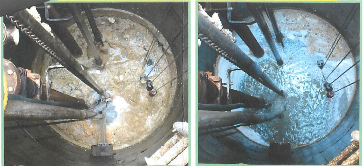
July 2017 photographs inside SLSA pumping station with FOG surface layer (left photo) and without FOG surface layer (right photo). This is ONLY the FOG that made it through the pipes. More could exist in the SLSA sewer pipes and your home's service line!
